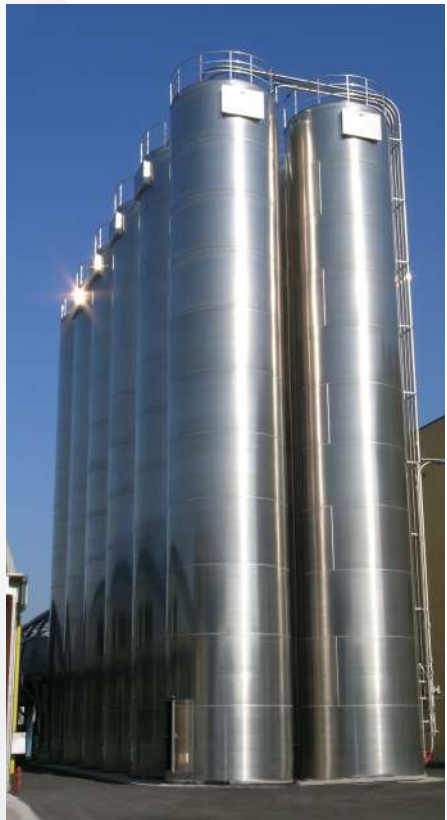
Silo with silo feeding system
